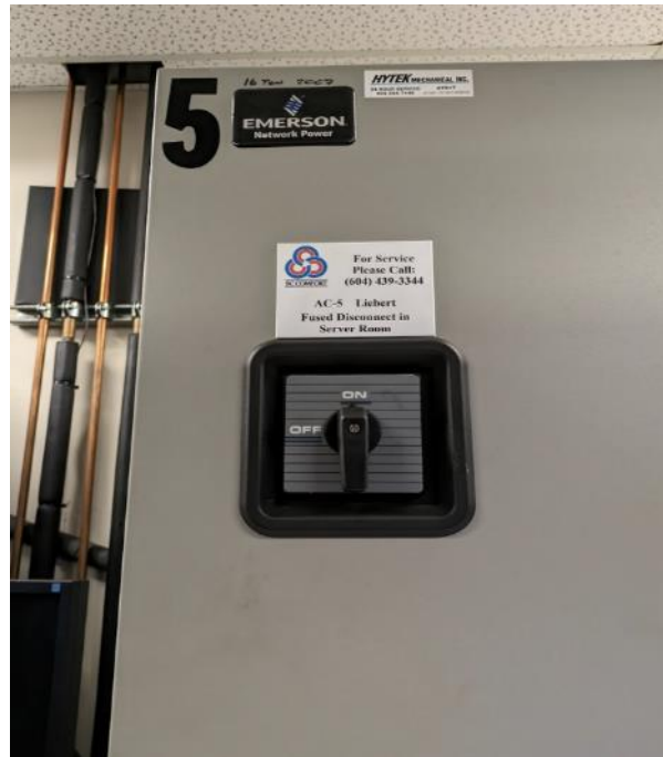
Figure 3.5: Mechanical cooling equipment and subfloor venting
