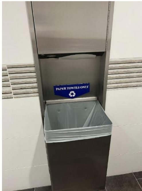
Figure 3.10: Representative paper towel receptacle bin in the bathroom.
